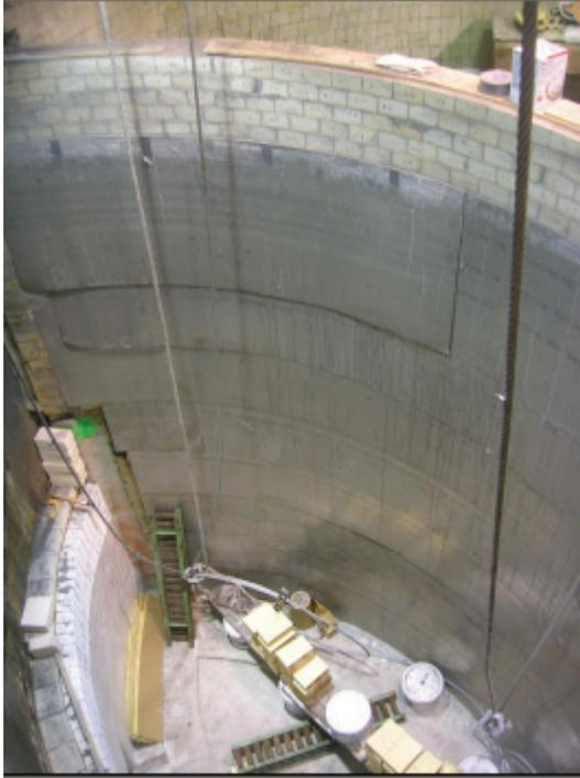
Figure 6: Gas Tight Barrier in Combustion Chamber wall.
