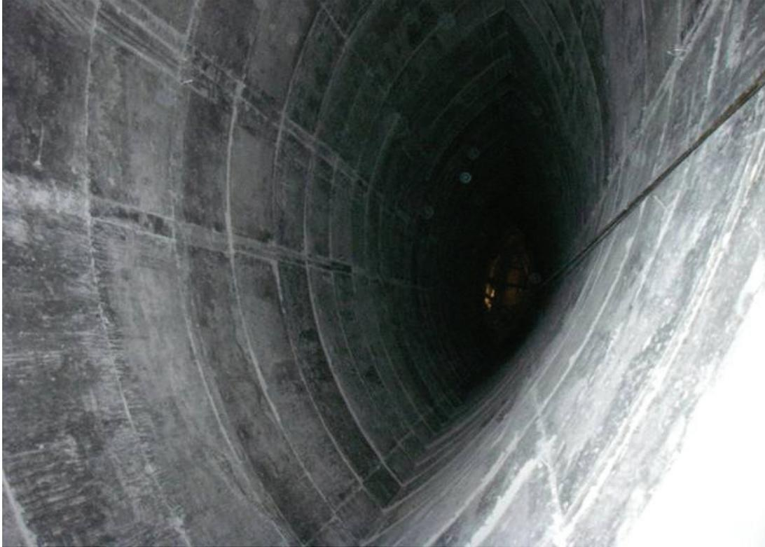
Figure 7: The Castable Combustion Chamber
